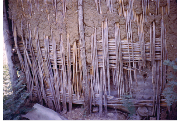
Figure 7. The detail of masonry bond of traditional Huğ House, 1998
