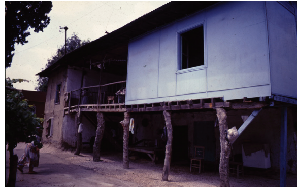
Figure 18. Two-storey Huğ House, Adana, 1999
