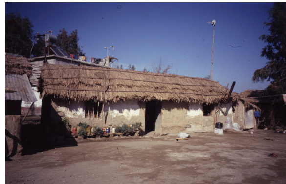
Figure 12. One-storey Huğ House wall and roof covering, Adana, 2000
