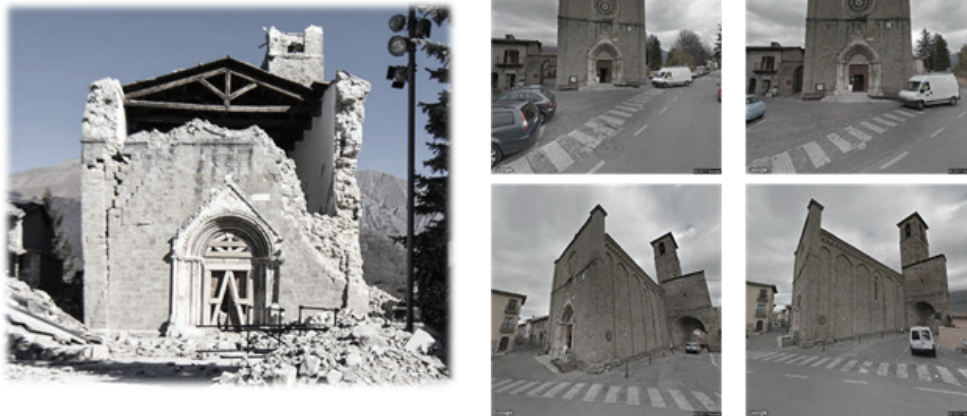
Figure 16. On the left we see the church of S. Agostino of Amatrice after the first shock, on the right a sequence of images that show the church today in Street View.
