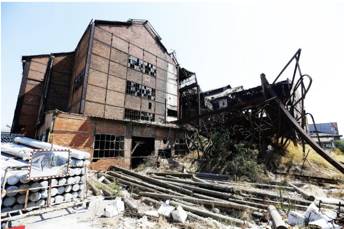
Fig. 20. Southern elevation of the factory in its current physical state.
