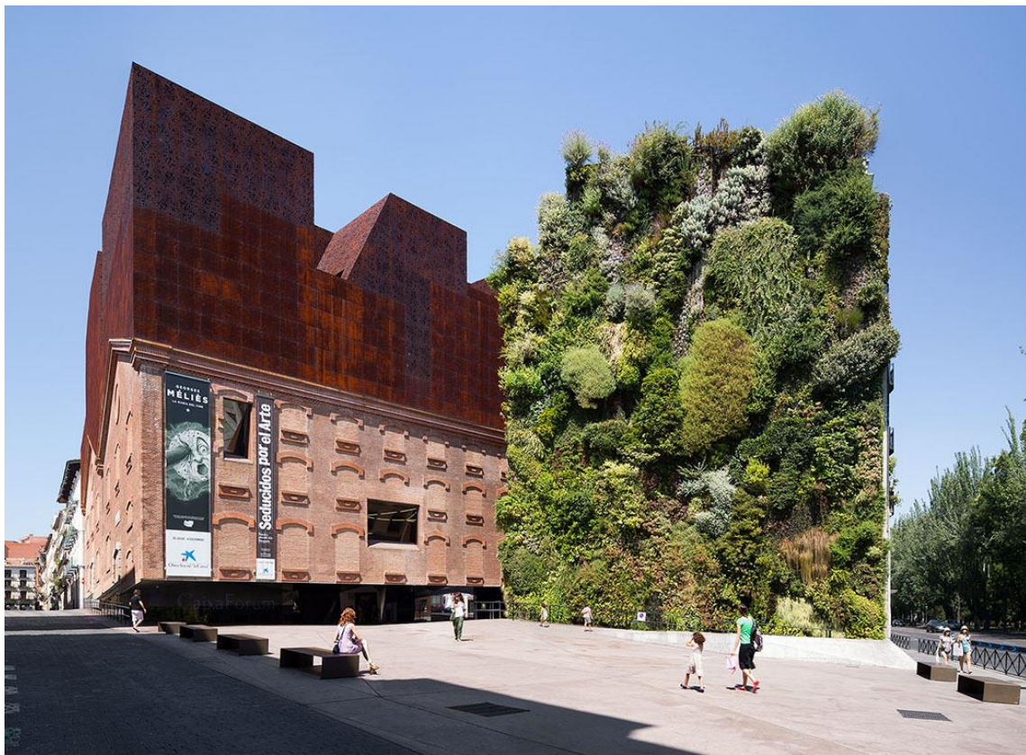
Fig. 2. External view of the Caixa Forum in Madrid, Spain.
