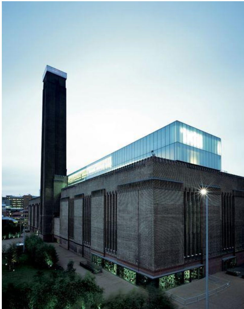
Fig. 7. External view of the two-storey Light Beam on the rooftop of the Tate Modern.
