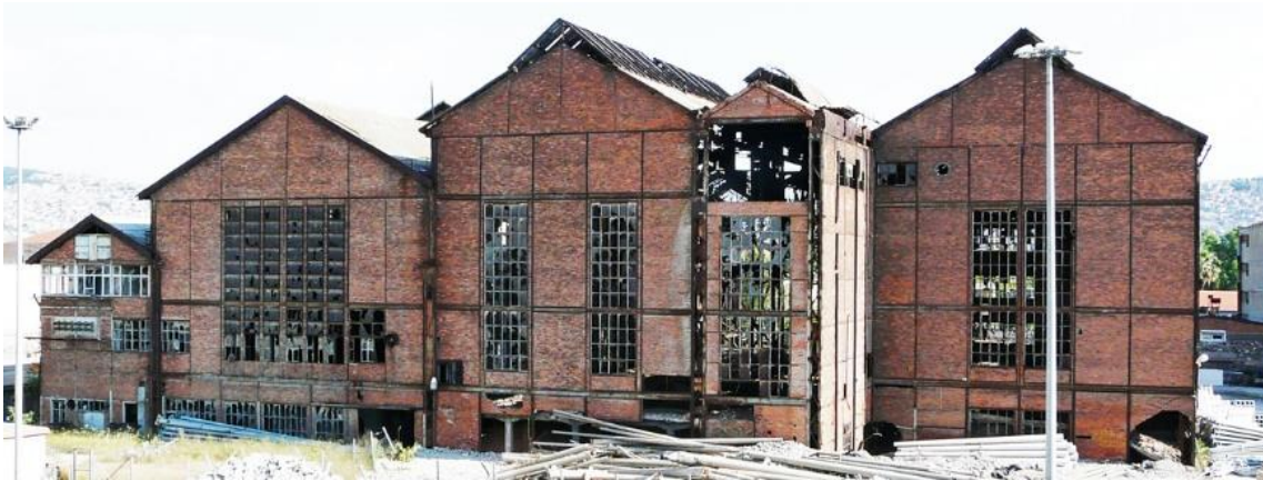
Fig. 19. Northern elevation of the factory in its current physical state.
