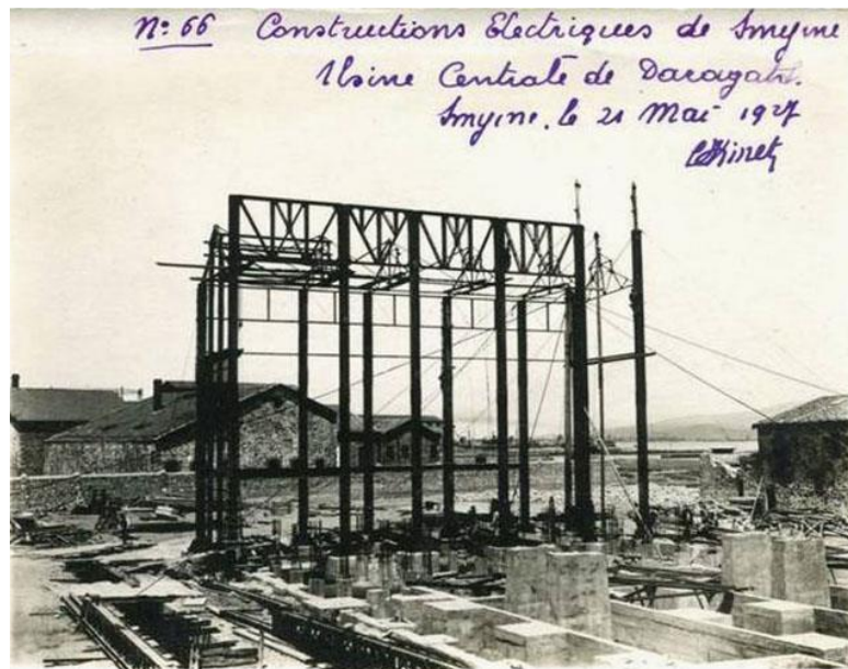
Fig. 18. Image taken during the construction of the Electric Factory in 1927.
