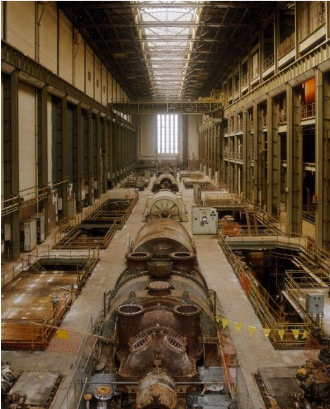
Fig. 4. View of the turbine hall of the Bankside Power Bank in the found state of the interior space before the adaptive reuse process for the transformation of the building into the Tate Modern.
