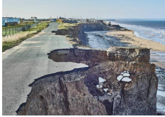
Fig. 5. Coastal erosion at Skipsea on the East Yorkshire coast.
